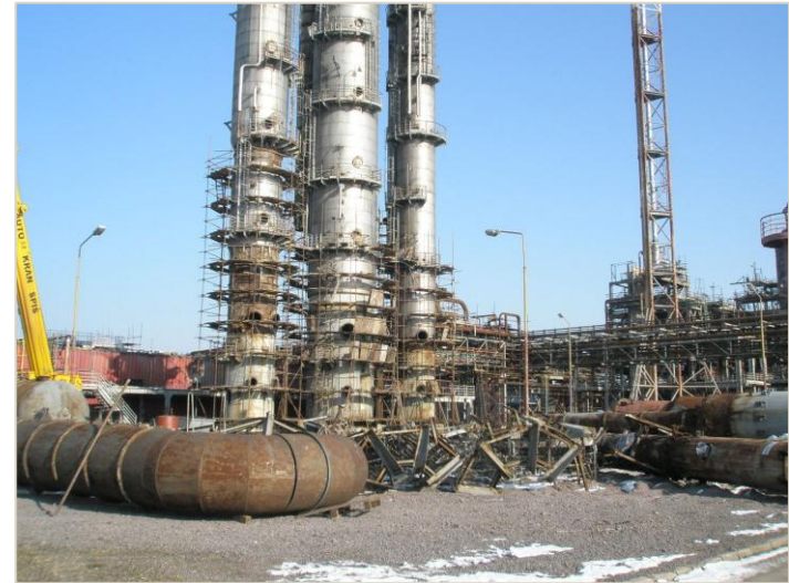
FIG. 10 – Cyclohexanone plant at Strážske during dismantling, 2009
