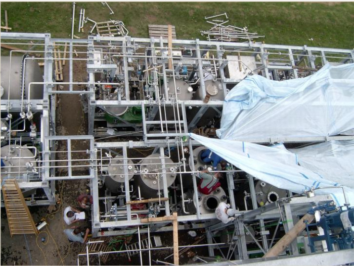
FIG. 09 – ENERGEA biodiesel plant modules during assembly, before shipment to Australia, 2006
